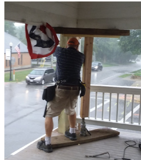
Orndorf Bracing Corner
