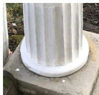
Rebuilt Pillar Base - 2023
