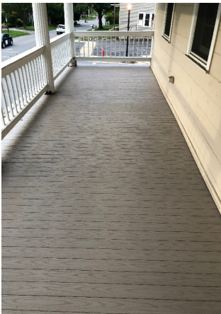
New Floor Complete
