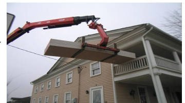
Porter donates and installs drywall
