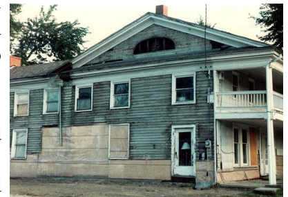
Sill replaced, siding & windows next
