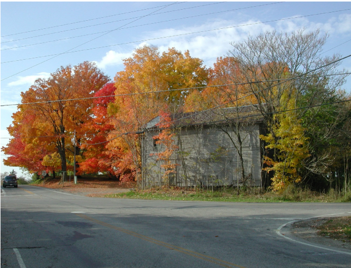
6340 St. Rt. 656 - Waiting To Be Torn Down
