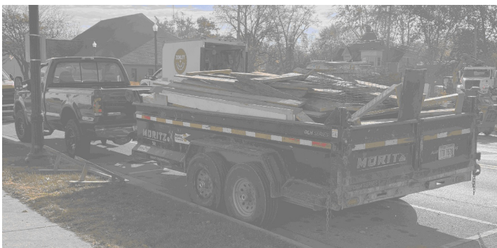
Filled Dumpster Ready to go
