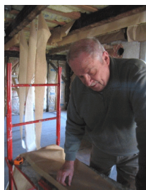
Joe (and Bess) Heiberger paper cover beams
