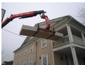
Porter Donates & Installs Drywall
