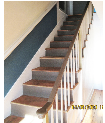
Finished stairway on April 5
